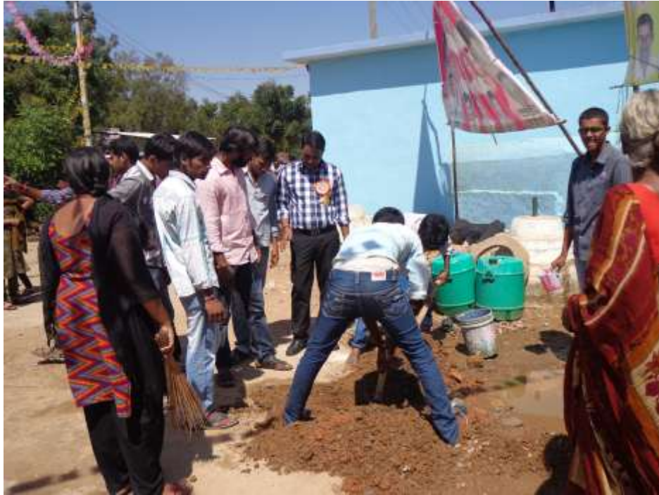
water pipeline repair
