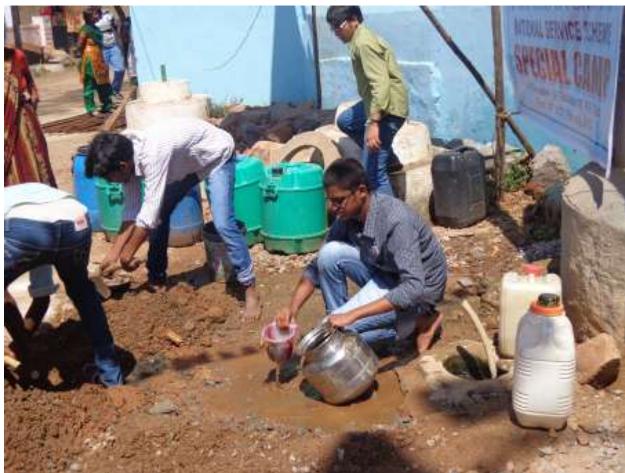
Clearing Drainage and waste water
