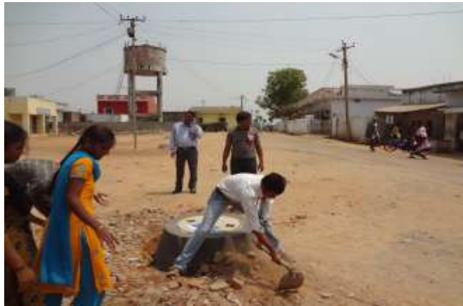
Levelling after waste clearance
