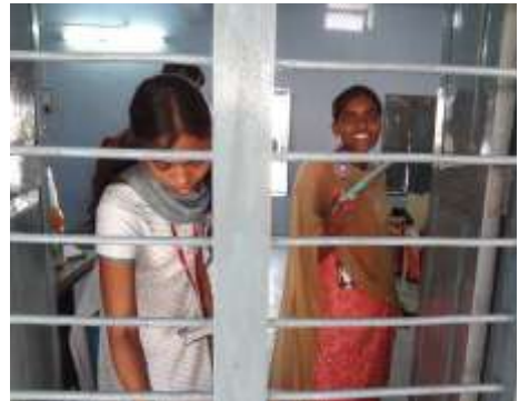
Painting the windows and grills
